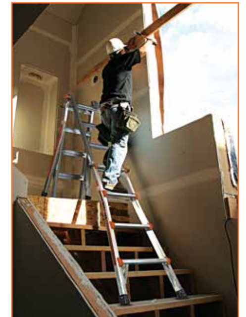
Safe, easy stair access.
