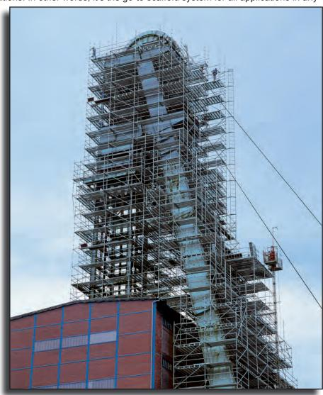
Scaffold for complicated structures like this pit head lift tower doesn't have to be complex. In fact, the Ring Lock system is engineered with only four basic components, so assembly is simple and quick.
